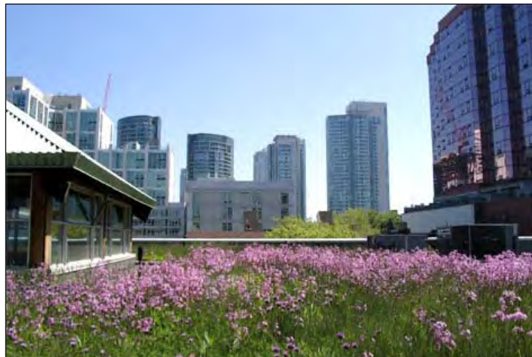
Green Roof on MEC's Downtown Toronto Store
