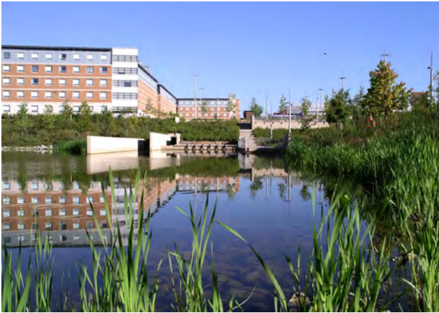
South Pond - UIOT Durham Campus (Oshawa, ON)
