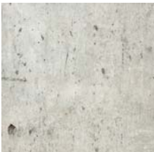
Concrete bench base
