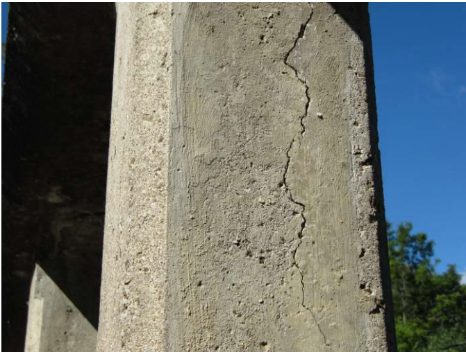
Plate 19: Detail of former patch-up work.
