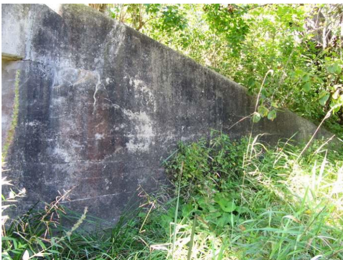
Plate 11: Detail of northwest wingwall.
