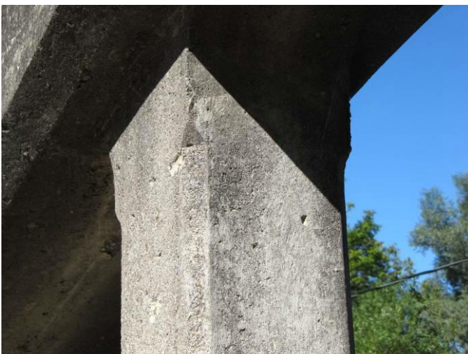
Plate 17: Detail of chamfered edges.
