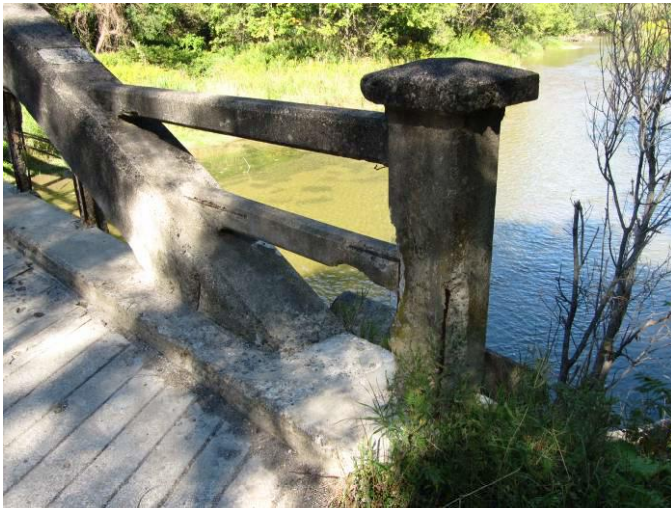
Plate 15: Detail of handrail and end post.
