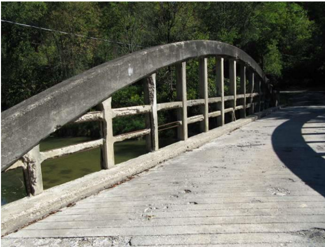
Plate 13: View of the north truss.
