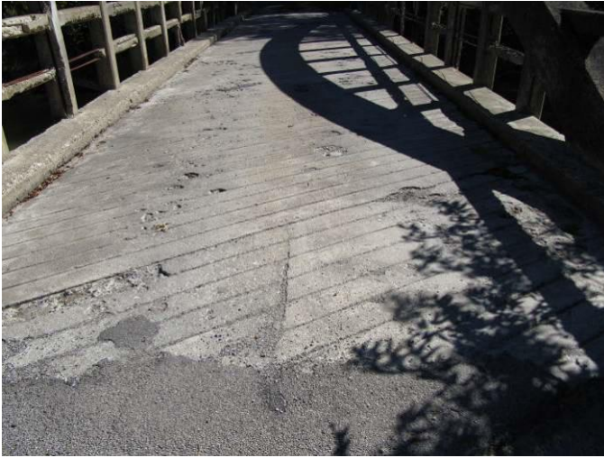
Plate 12: View of the bridge deck.
