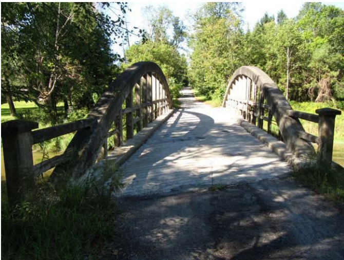
Plate 2: View of bridge crossing from the east.
