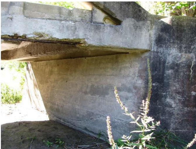
Plate 10: View of west abutment from the north.
