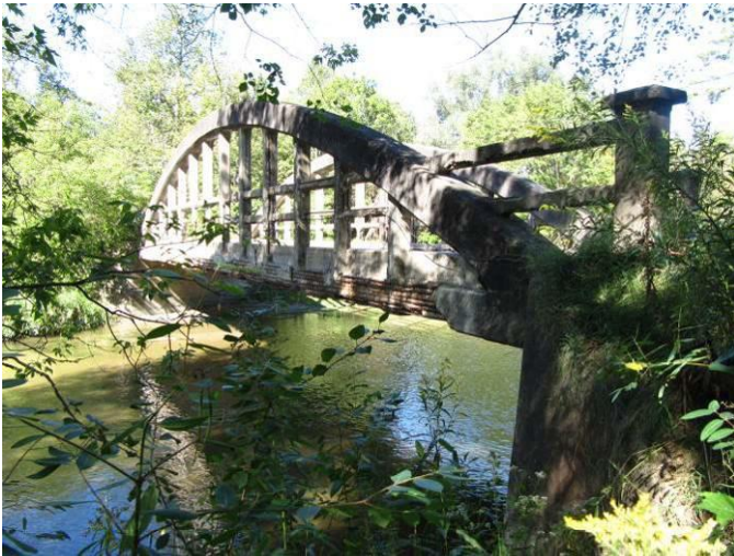
Plate 4: Oblique view of south elevation from the east bank.
