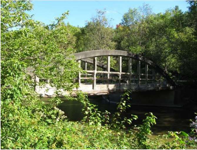
Plate 3: View of south elevation from the west bank.
