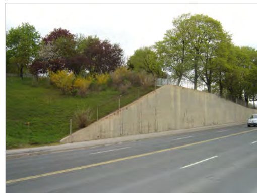
Concrete retaining wall east of railway bridge
