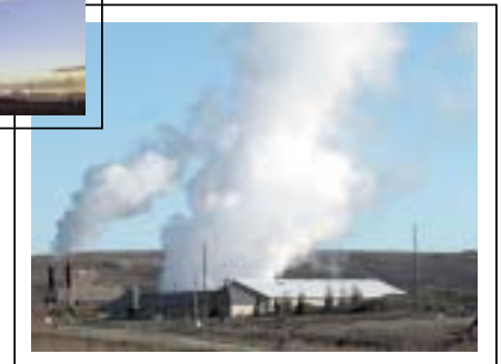
A POTENTIAL ENERGY SOURCE, A CLOUD OF STEAM IS RELEASED AT A NEARBY POWER GENERATION FACILITY CONNECTED TO A LANDFILL GAS COLLECTION SYSTEM.
