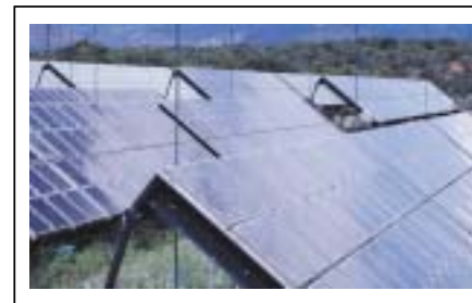
SOLAR POWER CAN BE DELIVERED USING VARIOUS TECHNOLOGIES, INCLUDING FLAT PLATE COLLECTORS TO POWER A BUILDING'S HOT WATER SYSTEM.
