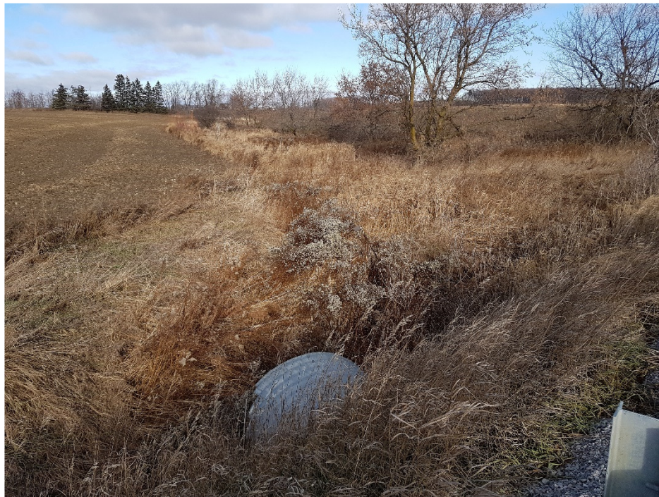
Photograph taken facing upstream (north) of Kirby Road. The swale feature flowed through an active agriculture field.
