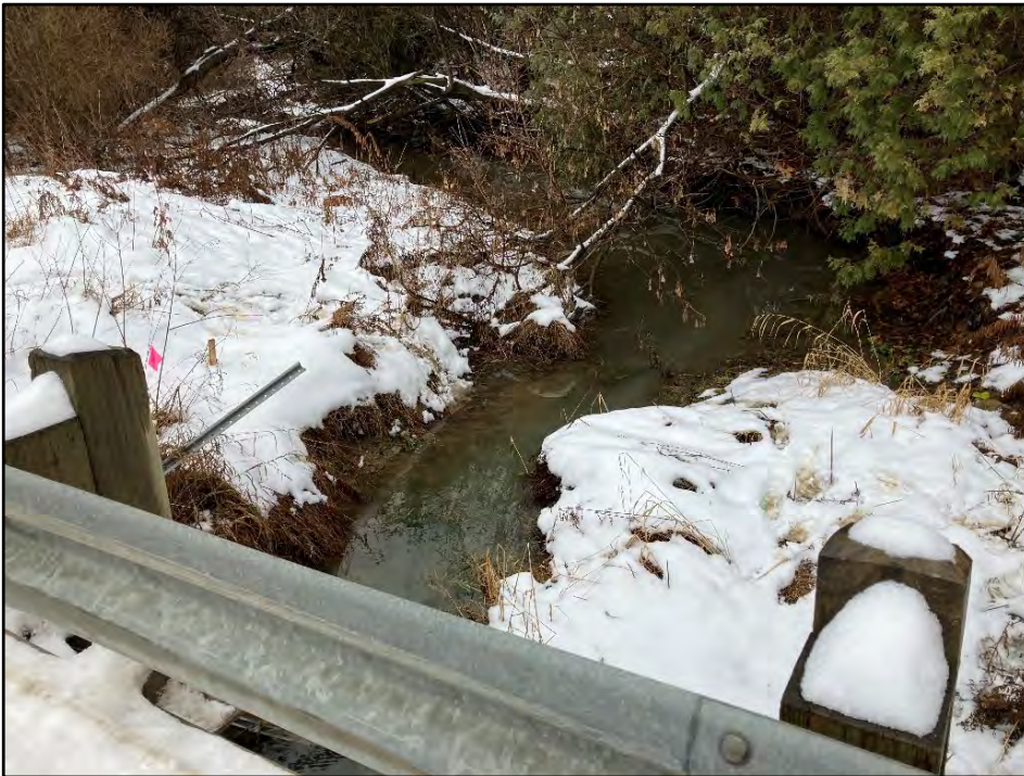
29. T2-R1 looking downstream from Teston Road crossing (Crossing 2). The channel is overwidened several meters downstream of the culvert outlet where it reaches a valley contact.
