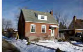
8233 Kipling Avenue + 1.5 Storey + Victory Housing, Circa 1950 + Red Brick + Single Central Dormer
