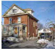
8255 Kipling Avenue Listed in VHI + 1.5 Storey + Gothic Revival, Circa 1870 + Whitewashed brick + Central Gable + Decorative Vergeboard + Edwardian alterations at grade
