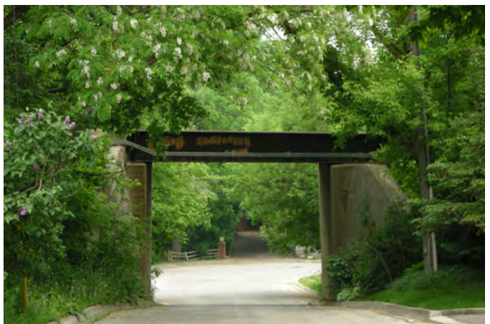
William Street - Rail Bridge
