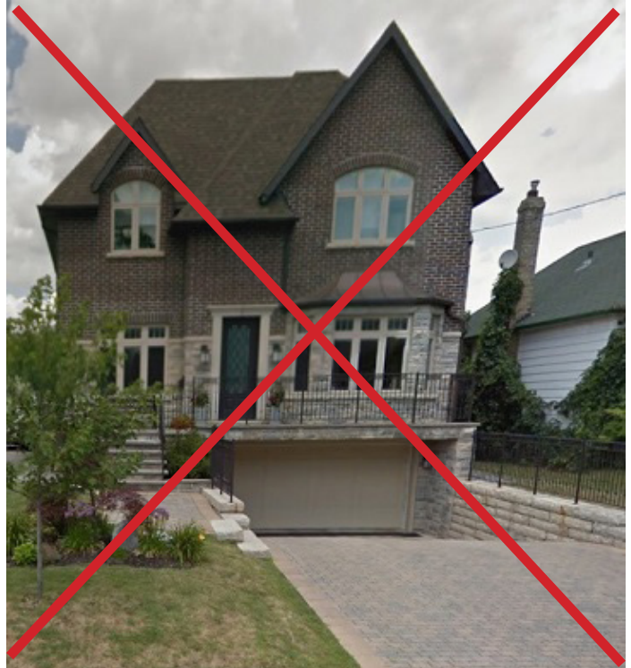
No portion of a garage should be located below the lowest grade of the lot at the street. (Guideline 4.20)
