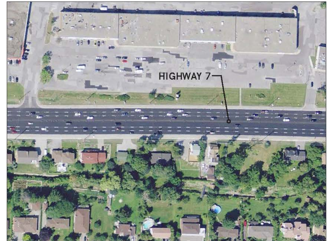
Figure 3.1.2 Aerial view along Concord West's existing Highway 7 corridor.
