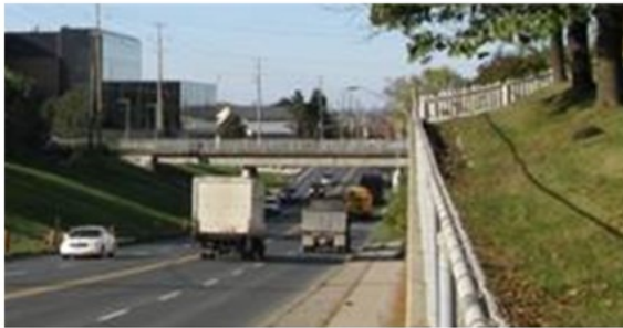
Underpass example on Major Mackenzie Drive east of Keele Street
