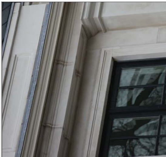
TYPICAL LIMESTONE FINISH UPPER WINDOW DETAIL
