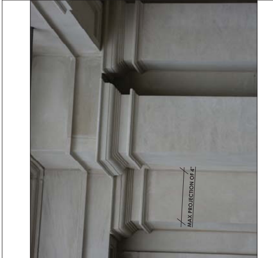
TYPICAL LIMESTONE FINISH PILASTER DETAILS
