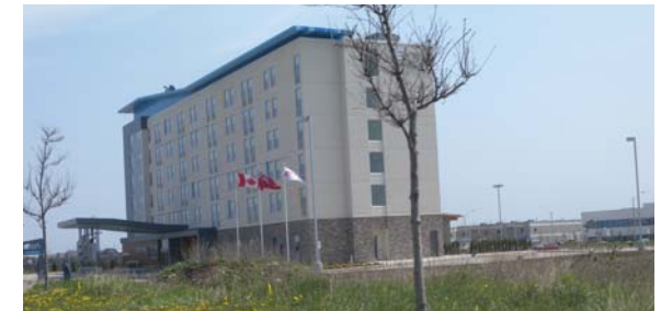
Recent hotel development in Vaughan Mills Centre
