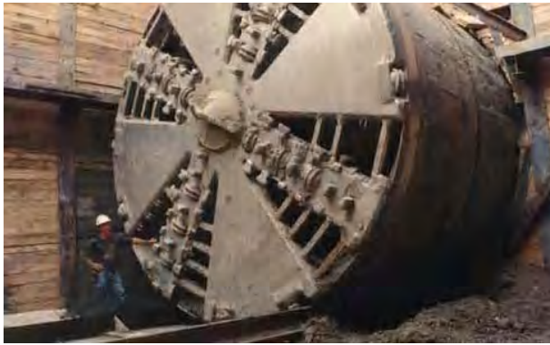
Head of tunnel boring machine; Sheppard subway construction
