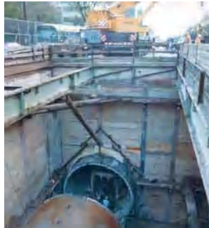
TBM in extraction shaft from Sheppard Subway
